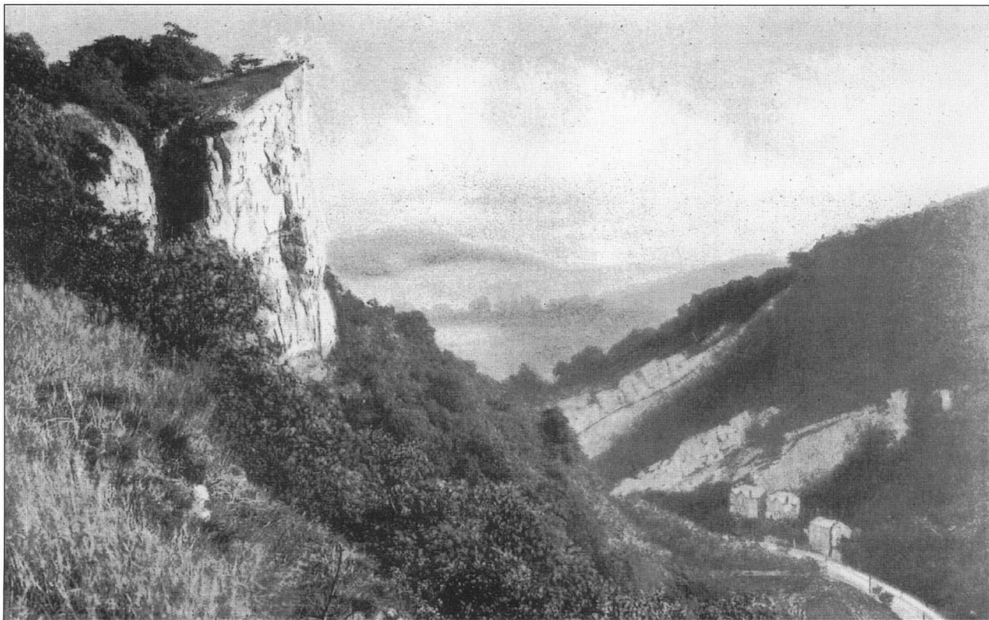
View southwards down the Gorge, taken from an old postcard of c.1900-1910. High Tor on the left with the mineral vein in the cleft. The two Long Tor quarries (hidden in trees today) show the dip of the Lower Matlock Limestones; the prominent partings are clay wayboards. The 1965 landslide destroyed the middle house and damaged the others.
